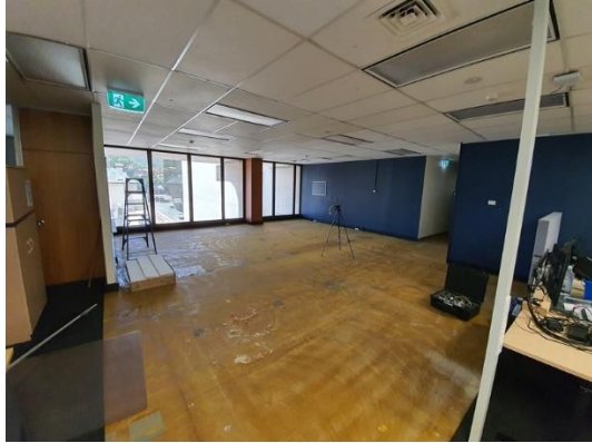
Image 5: 2 nd Floor affected area after remediation.
